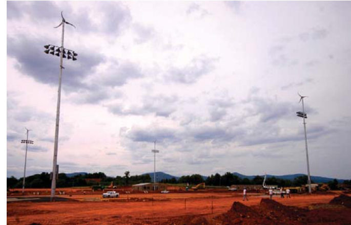
FLEMING STADIUM LIGHT TURBINES
