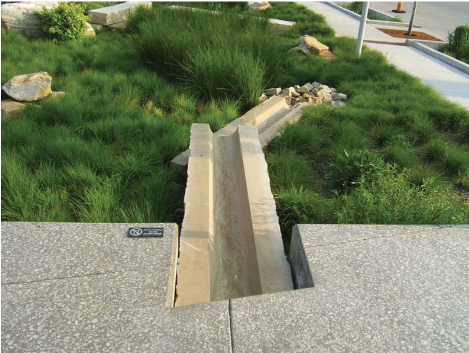
[Below] Rain garden by 360 Architects
