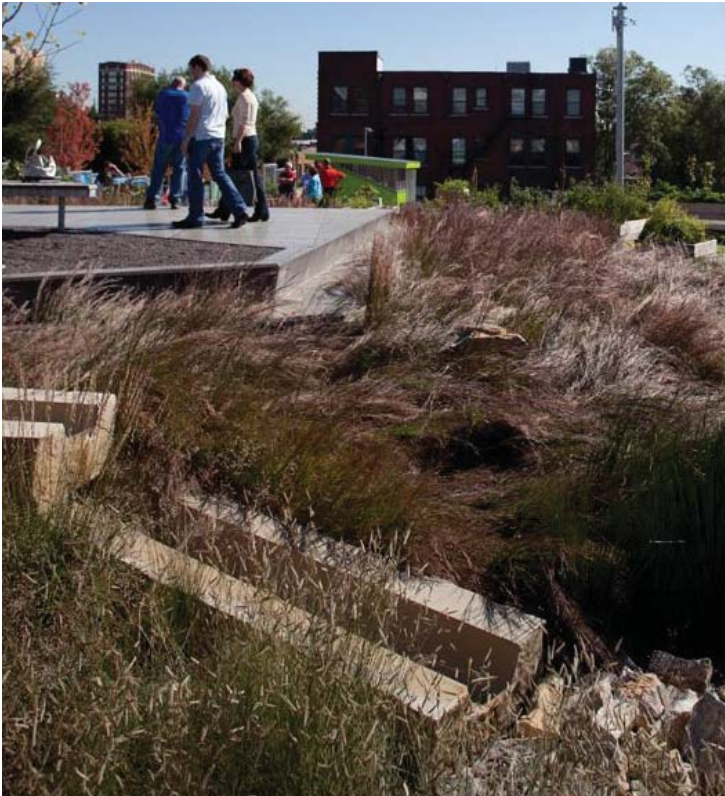
[Left] Biofiltration system cleanses and stores water to be reused for irrigation.
