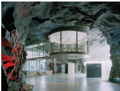
WHITE MOUNTAIN DATA CENTER
